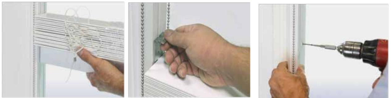
**Step 15** Raise the slat stack to within a few inches of the tilt rail and remove the shrink-wrap. Rotate the tilt rail backwards and attach the back ladders to the receptacles in the tilt rail. Then rotate the tilt rail forwards and attach the front ladders.
