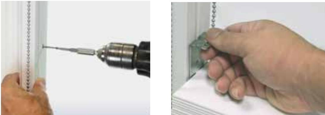
**Step 14** Raise the stack to just under the top screw hole, remembering to support the stack with your hand as you use the bead chain. Insert the gap gauge, pull the side guides snug, and then install the top screws.
