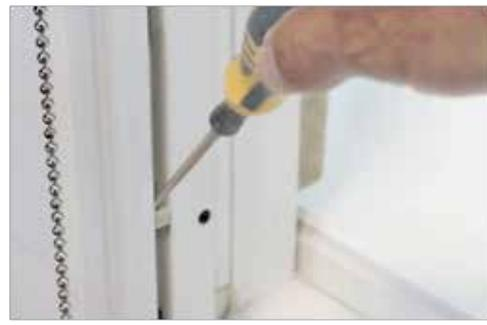
**Step 5** Position the lift side guide (the one with continuous outer bead chain) squarely in the opening and drill pilot holes through the existing countersunk holes in the side guide. Make sure that the side guide remains in the proper position while drilling. The pilot holes must be absolutely straight, as this will eliminate the possibility of a side guide being installed at an angle. Set the lift guide beside the opening within easy reach.
