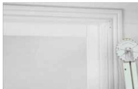
**Step 6** Position the tilt side guide squarely in the opening, drill the pilot holes and then install the middle screw. The screw threads will be used to make micro adjustments later so never bury the head, simply insert until head is flush with side guide surface.
