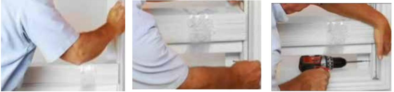
**Step 13** Use one hand to lift the stack while pulling down on the bead chain to raise the stack to halfway point, just beneath the middle counter bore holes. Back out the previously installed middle screw on the tilt side guide. Insert the gap gauge, pull the side guide snug to the gap gauge and center to the opening then install screws.
