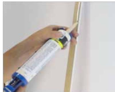
**Step 2** Place the trim strip on the inside edge of the opening flush with with the edge.
